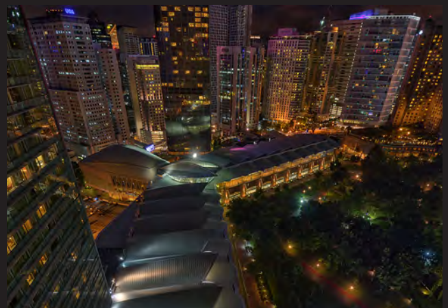
Kuala Lumpur Convention Centre - Malaysia
